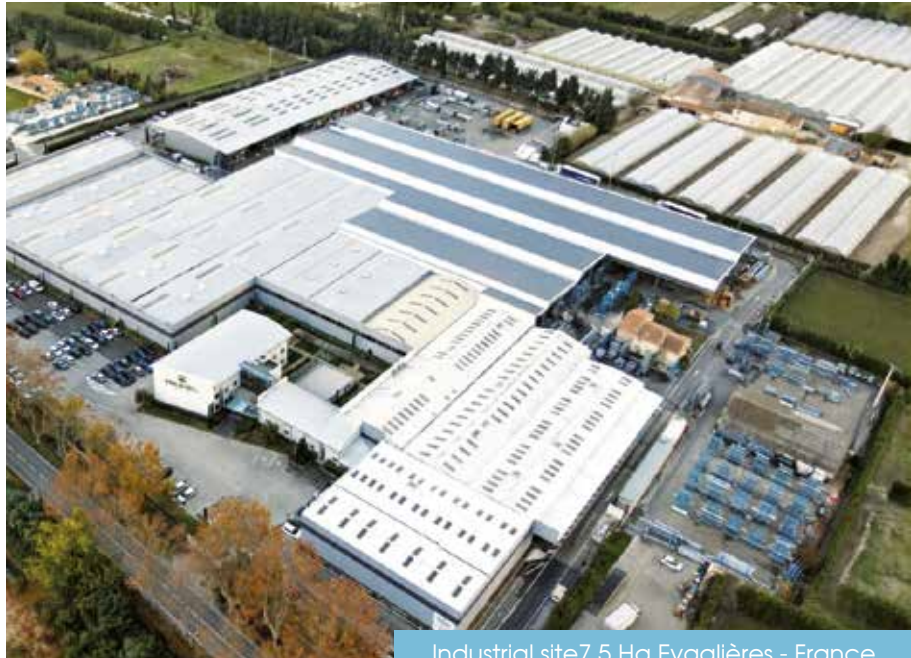
Industrial site 7.5 Ha Eygalières - France
